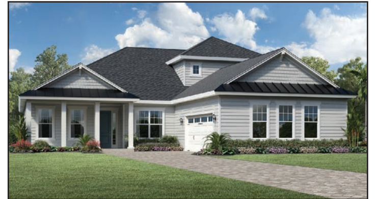
Photos provided by Beacon Lake
